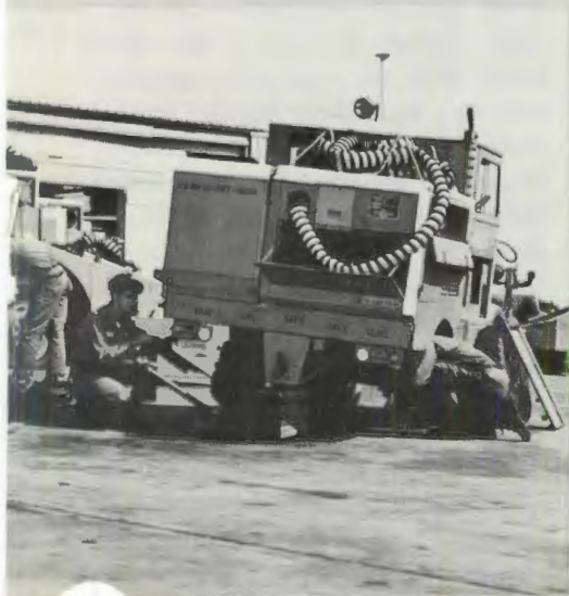
Personnel at work getting out-of-mission units back on the line.
